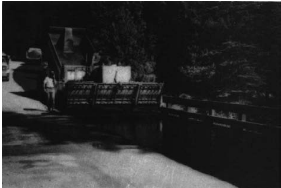
Figure 11-10. - Crushed aggregate chips are applied over an asphalt binder by a self-propelled aggregate spreader (photo courtesy of Paul Cole, USDA Forest Service).
