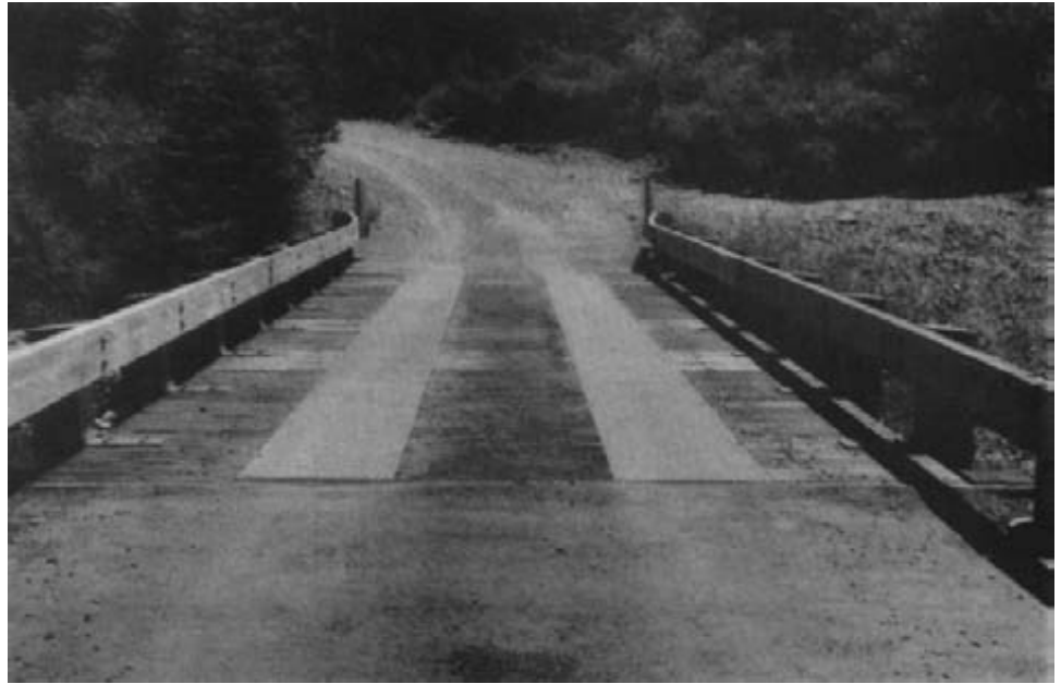
Figure 11-20. - Steel running plate wearing surface on a timber bridge deck.
