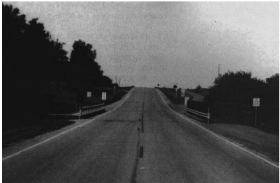
Figure 11-3. - Asphalt pavement wearing surface on a timber bridge deck.
