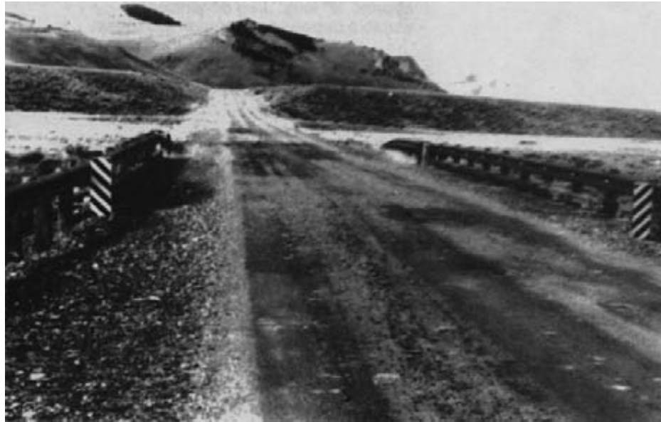
Figure 11-29. - Aggregate wearing surface on a timber bridge deck.
