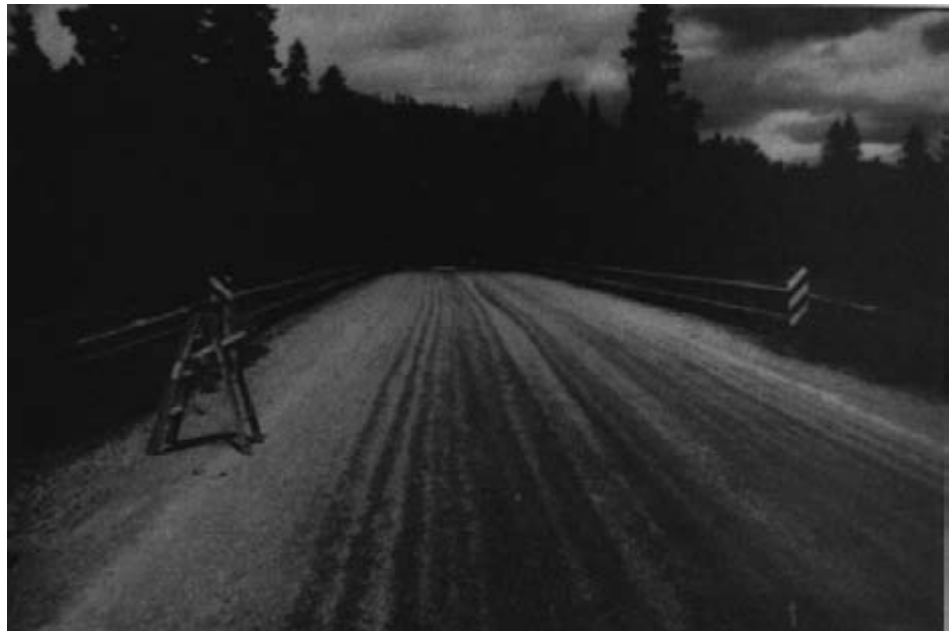
Figure 11-8. - Asphalt chip seal wearing surface on a timber bridge deck.
