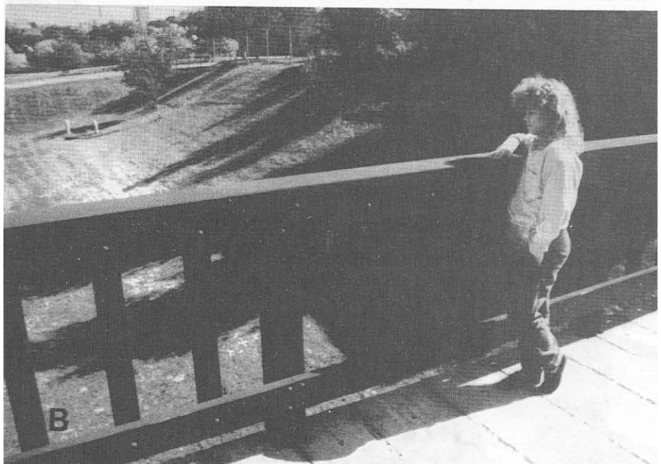
Figure 10-13. - Typical pedestrian/bicycle railing configurations used on timber bridges. (A) Glulam rails mounted on glulam posts. (B) Lumber posts with horizontal rails and vertical pickets.
