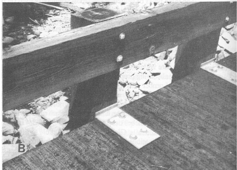
Figure 10-7. - Types of vehicular rails commonly used on timber bridges. (A) Glulam beams. (B) Sawn lumber beam.
