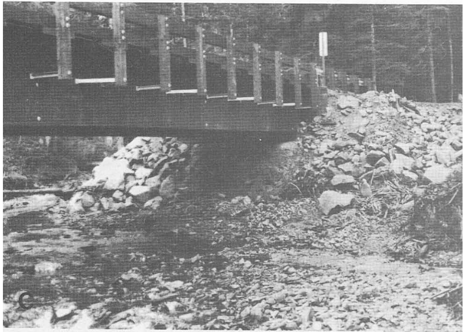
Figure 10-9. - Typical vehicular railing configurations used on timber bridges (continued). (B) Lumber posts attached to steel plates that are bolted through a glulam deck. (C) Lumber posts bolted to a lumber curb with braces attached to a glulam beam.
