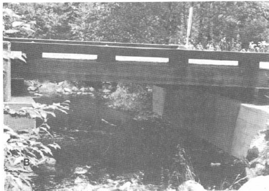
Figure 8-2. - Longitudinal glulam deck bridges. (A) Panel placement during construction of a multiple-span bridge. (B) Typical single-span bridge configuration (photo courtesy of Dave Nordenson, USDA Forest Service).
