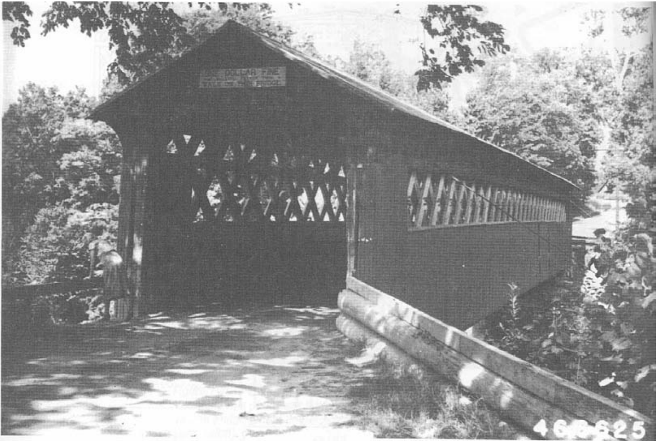
Figure 1-13.-Typical Town lattice truss covered bridge.
