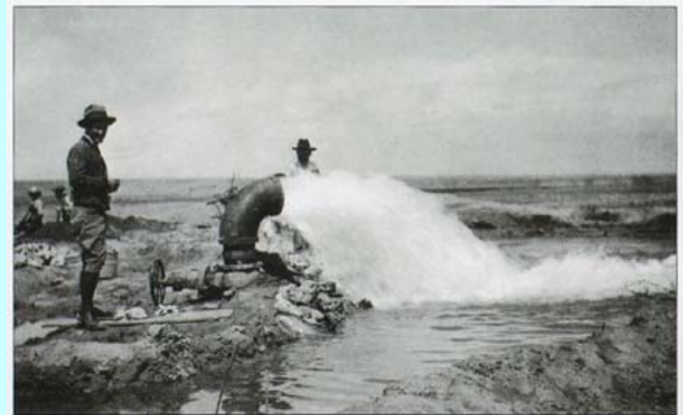
Figure 100. This flowing well was completed in the carbonate-rock aquifer 8 miles southeast of Roswell, N. Mex. On April 21, 1926, it flowed at a rate of 3,190 gallons per minute.
