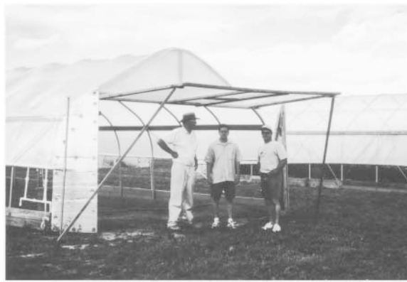
Fig. 13. Center section of lower portion of the end walls used in the Penn State high tunnel design opened up to allow easy entrance and exit of machinery.
