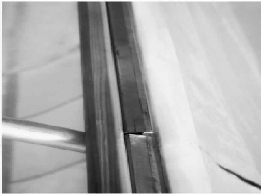
Fig. 6. Surelock aluminum double-rail track attached to the hipboard used to attach the plastic covering to the top and side of the high tunnel. Clip is being fastened to the lower track.
