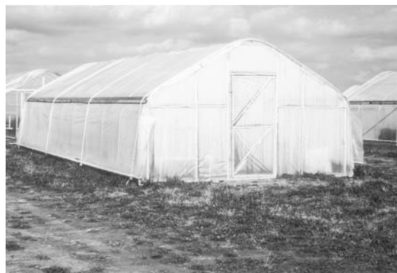
Fig. 1. High tunnel constructed using the New Hampshire design developed by Otho Wells, University of New Hampshire.
