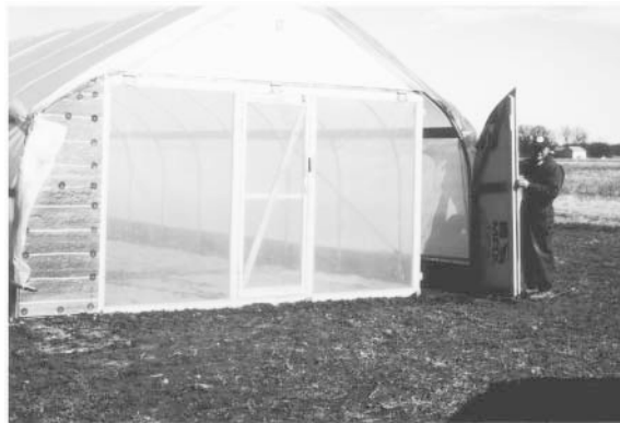
Fig. 14. Side panel opened up before raising the center section in the Penn State high tunnel design.
