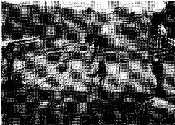
Figure 7—Application of waterproof membrane.
