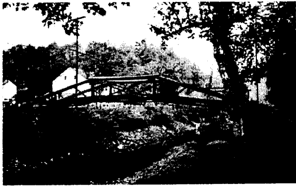
Figure 6-Original Camelback Truss Bridge
