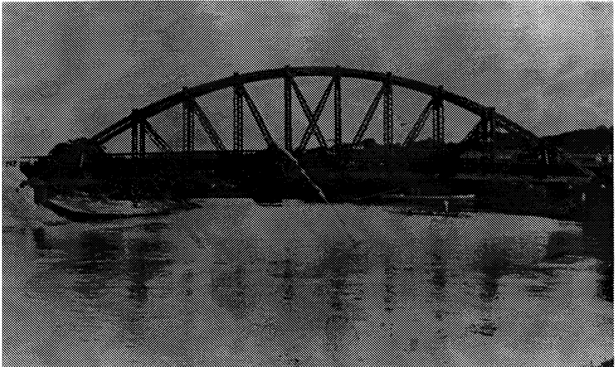
Figure 8. Bowstring truss bridge over Tiete river. This bridge was 52 meters long, consisted of two longitudinal bowstring truss beams of Peroba Rosa specie and was built in 1930.
