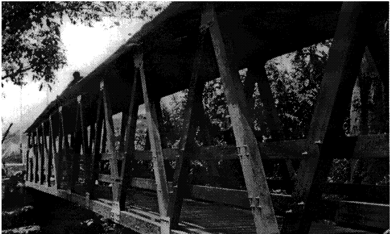
Figure 9. Parallel chord truss bridge over Chinchina river, Colombia. This bridge was 30 meters long, consists of two longitudinal parallel truss beams of Culiferro specie and was built in 1987.
