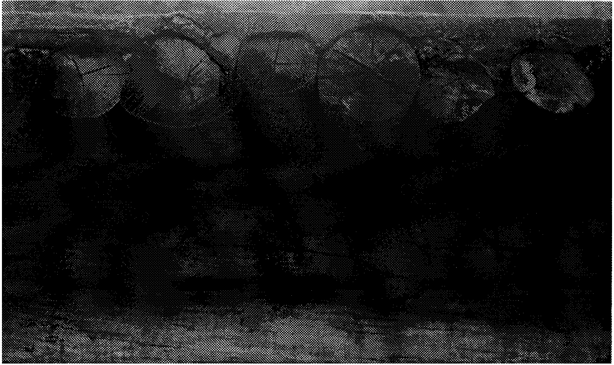
Figure 14. Composite logs-concrete deck attached to longitudinal beams with steel strip and lag screws.
