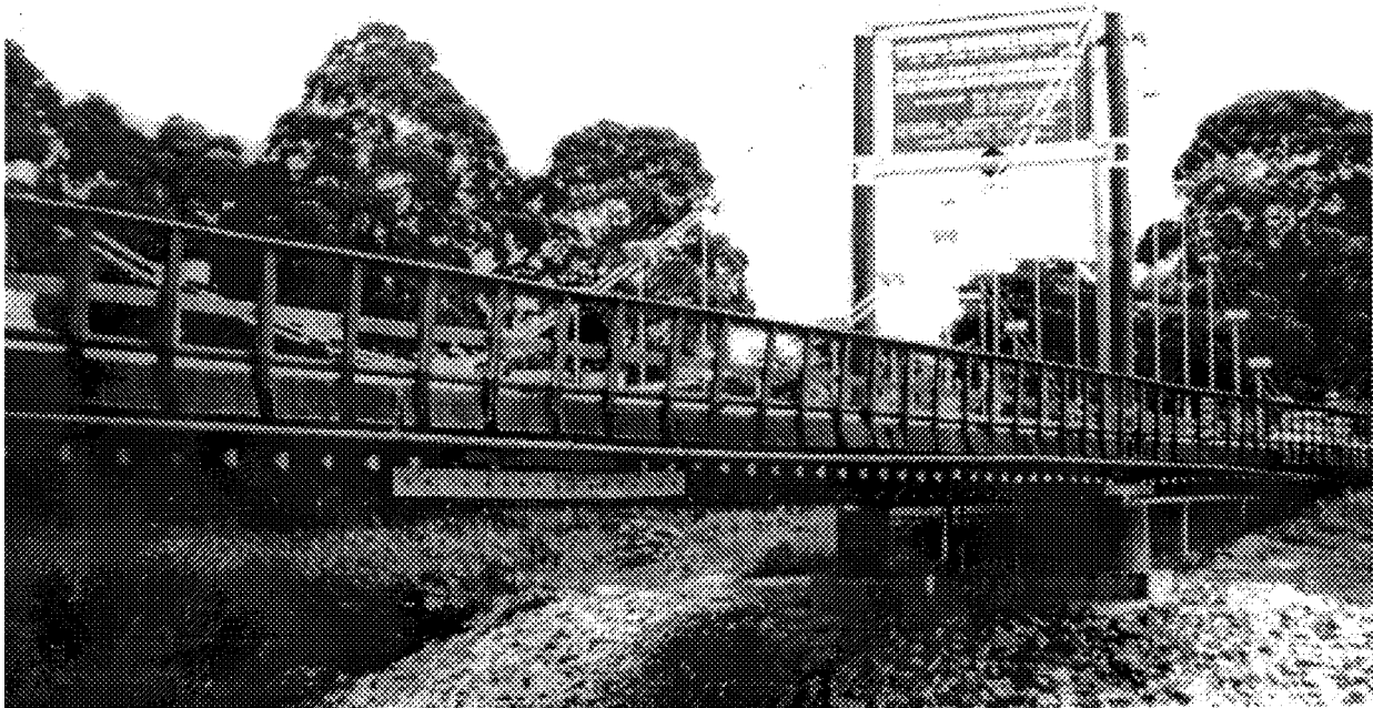
Figure 16. Suspnsion bridge over Tiete river. This bridge is 62 meters long, 31 meters span, consists of two longitudinal composite log beams of Eucaliptus specie, was designed by LaMEM in 1977.
