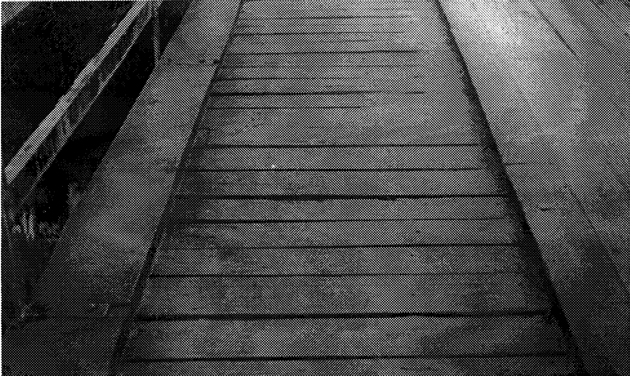
Figure 11. Transverse sawn lumber plank deck attached to longitudinal beams with spikes.
