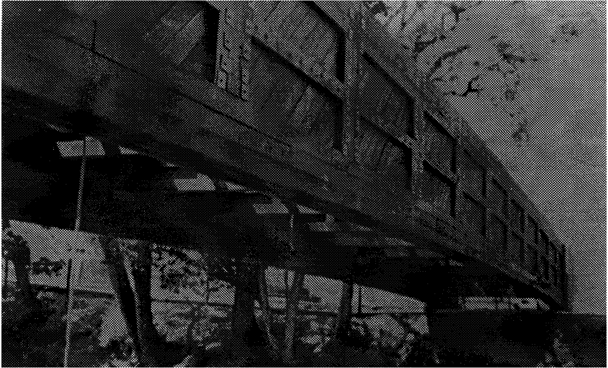
Figure 7. Multi-lattice boarded nailed system over Sorocaba river. This bridge is 28 meters long, consists of two longitudinal nailed I beams with diagonally crossed web of Macaranduba specie and was built in 1990.
