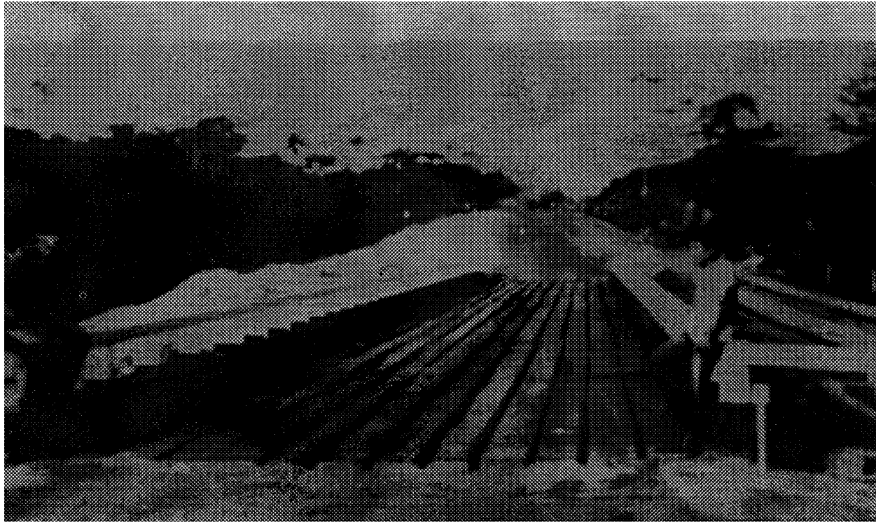
Figure 12. Longitudinal sawn lumber plank deck attached to longitudinal and transversal beams with spikes.
