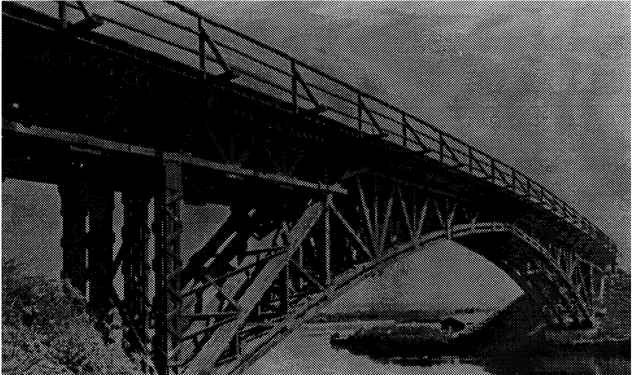
Figure 10. Strut frame truss bridge over Tiete river. This bridge was 60 meters long, consists of four longitudinal strut frame truss beams of Peroba Rosa specie and was built in 1930.
