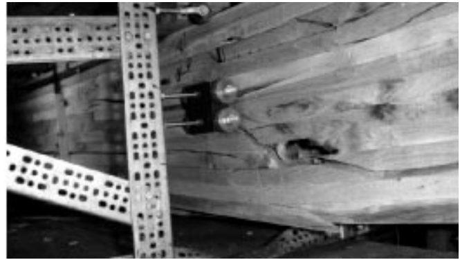
Figure 5—Rupture of a beam at ultimate load through the three E-rated laminations on the tension side and into the No. 3 grade inner laminations.
