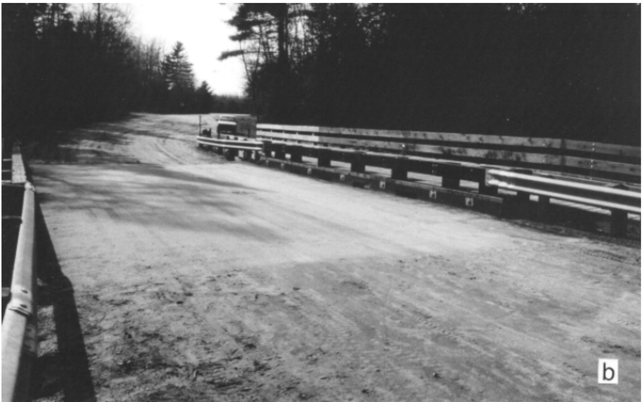
Figure 11—Completed Graves Crossing bridge: (a) side view, (b) end view.
