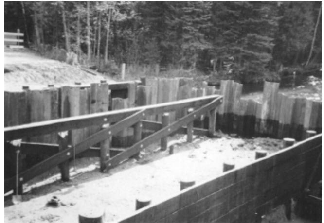
Figure 4—Coffer dam used during installation of timber piling, abutments, and bent.
