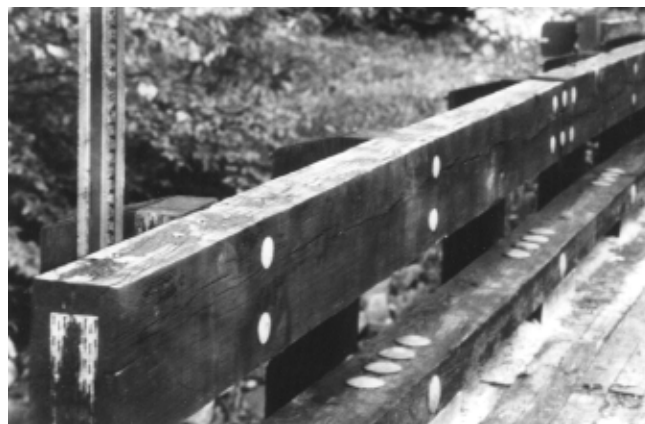
Figure 13—Spiked metal plates in the end grain of sawn lumber curb and rail members.
