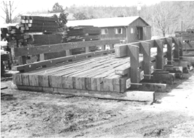
Figure 2—Prefabricated stress-laminated bridge deck at the fabrication facility.
