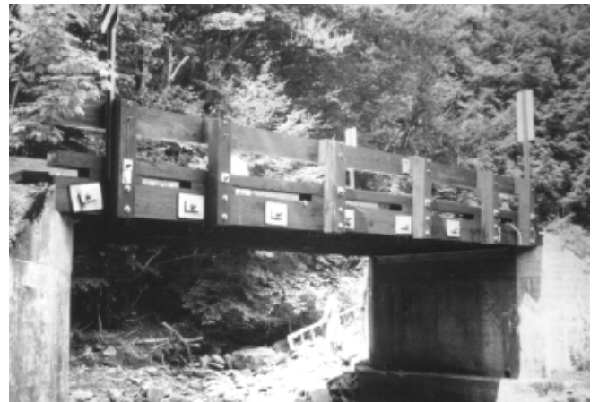
Figure 7—Completed bridges: Birchlog Run bridge, (top) Tumbling Rock Run bridge (bottom).
