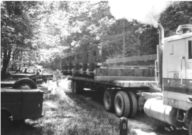
Figure 3—Delivering bridge deck to the construction site on a tractor trailer.
