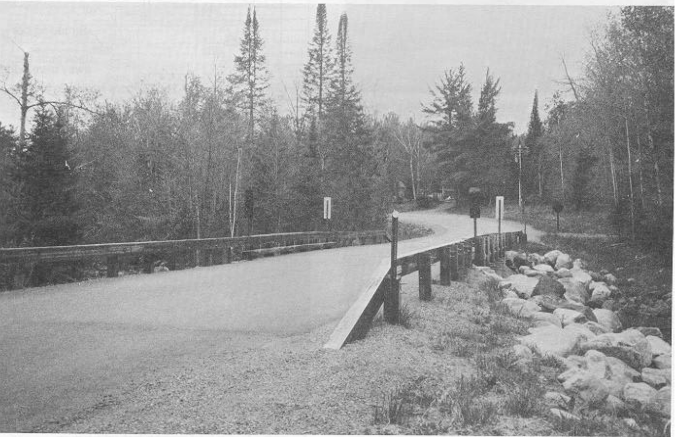
Figure 9—Completed Teal River bridge. (M92 0001-26, M92 0001-24)
