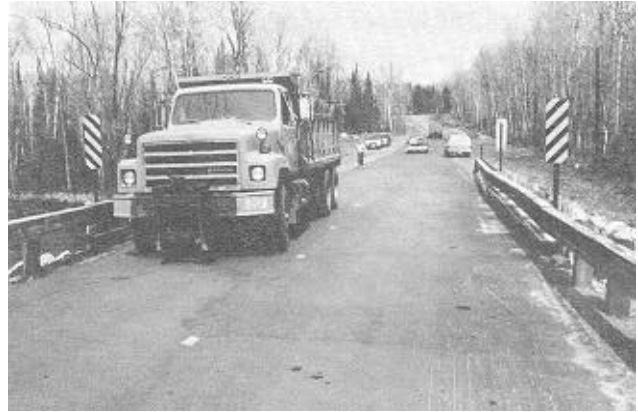
Figure 18—Load position 2 with a single vehicle in the upstream lane. (M92 0009-12)
