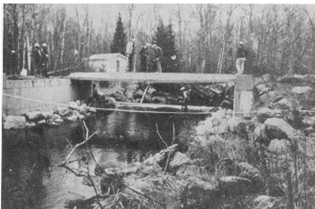
Figure 6—Placement of beam laminations on abutments. (M92 0009-4)
