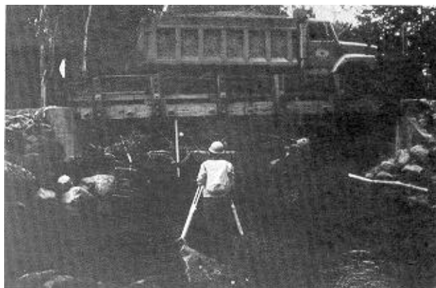
Figure 15—Measuring bridge deflection with surveyor's rod. (M92 0009-9)
