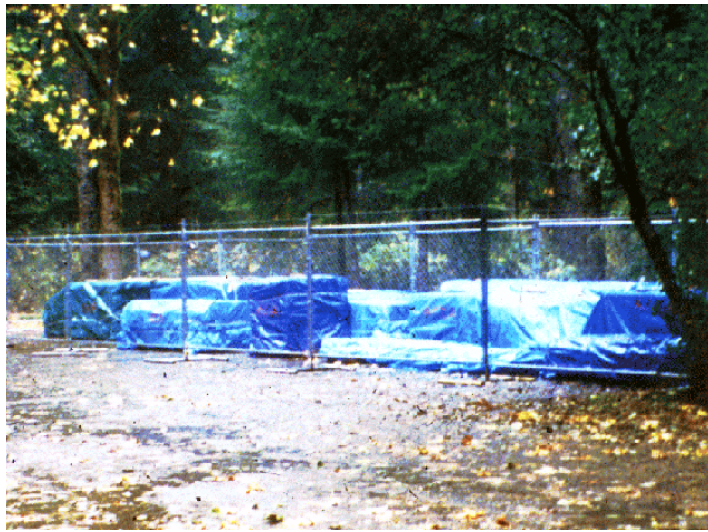
Figure 4—Treated lumber delivered for construction projects should be supported off the ground and covered.
