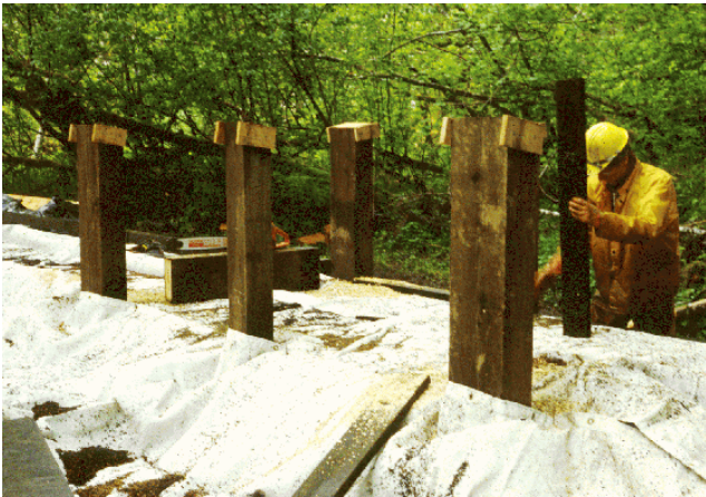
Figure 8— Tarps can be used to contain and collect sawdust generated during on-site fabrication.
