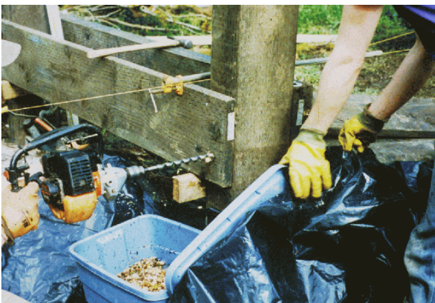
Figure 9— Plastic tubs are useful for collecting shavings when boring holes on-site.
