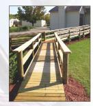
ACCESSIBILITY RAMP: Our new access ramp is also a durability project using nine different preservative-treated woods, four wood-plastic composite materials, and three naturally
