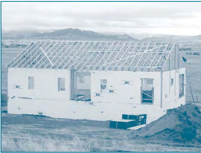
An ENERGY STAR-qualifying home under construction in Montana.
