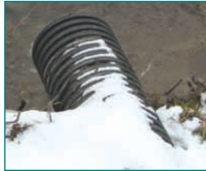
Freezing is unlikely to be a concern, as soils rarely freeze as deep as the tile.
