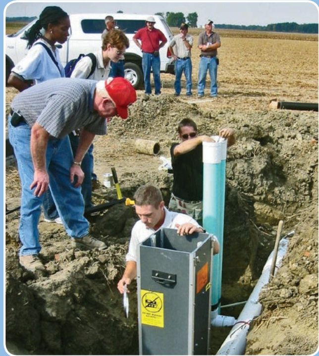
Installing structures to help control subsurface drainage.
