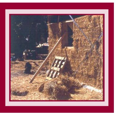
sible to finish interiors with gypsum wallboard and exteriors with different siding options. In some agricultural buildings owners have left bale walls unfinished, recognizing that this leaves them vulnerable to damage from livestock and weather.
