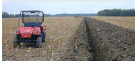
A new tile drain in Ohio
