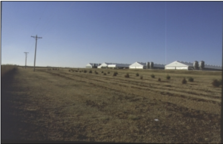
Figure 8. Planted in April 1999, this five row mixed conifer and hardwood species shelterbelt is located on the northwest corner of a swine confinement facility in central Iowa. This shelterbelt was planted specifically for odor control and improved aesthetics. Photograph by A. Holtz, Iowa State University, 1999.
