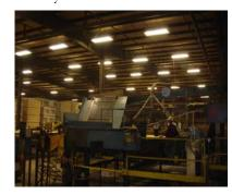
fixtures and fixtures containing standard T12 fluorescent lamps and magnetic ballasts. Metal halide lamps were left on continuously and fluorescent fixtures were turned off only sporadically.
