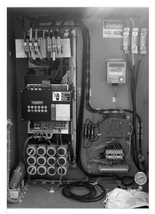
This variable frequency drive ensures the irrigation pump will operate at the right speed for the size of the job, saving energy.
