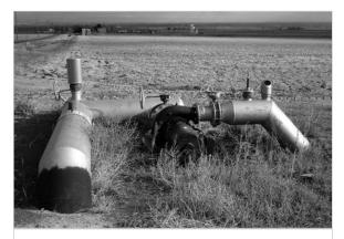
A variable frequency drive controls the speed of this efficient pump in Malheur County, saving electricity.
