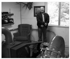
Lucien Gunderman stands behind two turbines in the main hydroelectric facility. The turbines have a combined capacity of 30 kilowatts.
