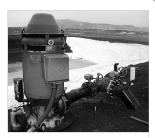
A variable frequency drive controls the speed of this irrigation pump in Union County, saving electricity.
