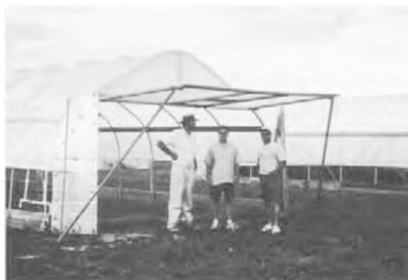
Fig. 13. Center section of lower portion of the end walls used in the Penn State high tunnel design opened up to allow easy entrance and exit of machinery.
