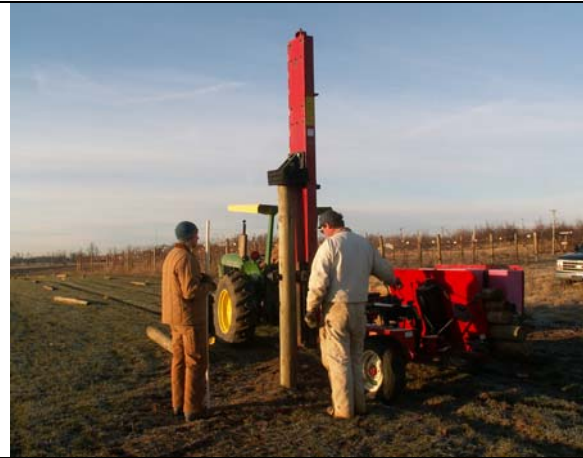
Figure 2. Driving in posts at marked locations
