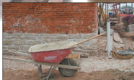
Above and clockwise: West side of the 1819 Hickman House, currently under restoration. The original stone foundation at the Hickman House was recently reinforced with concrete in 4-foot sections. Cracks in the original interior plaster reveal brick walls. Original log floor joists are uncovered.
