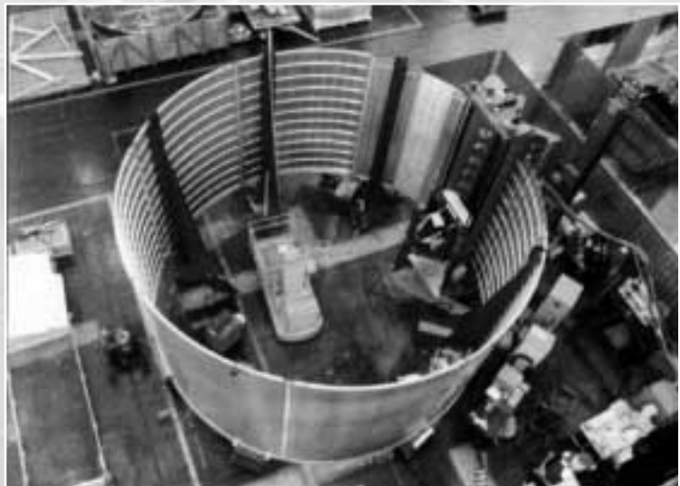
Friction Plug Welding Repair
