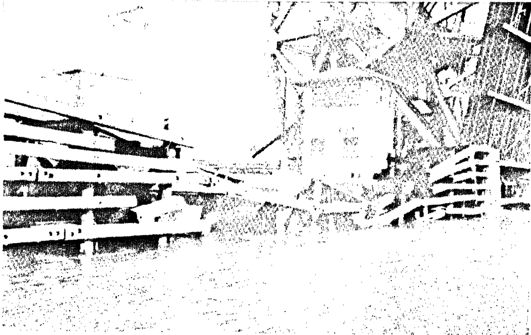
A NEW ORLEANS INNER HARBOR NAVIGATIONAL CANAL BRIDGE WITH AN EXTENSIVELY DAMAGED PIER PROTECTION SYSTEM.
