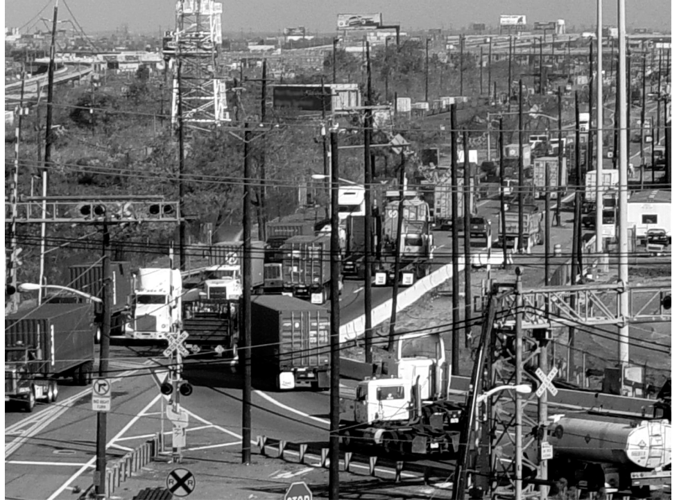
Figure 4: Connector to the Elizabeth New Jersey Port Authority Marine Terminal: Intersection of North Fleet Street and Corbin Street
