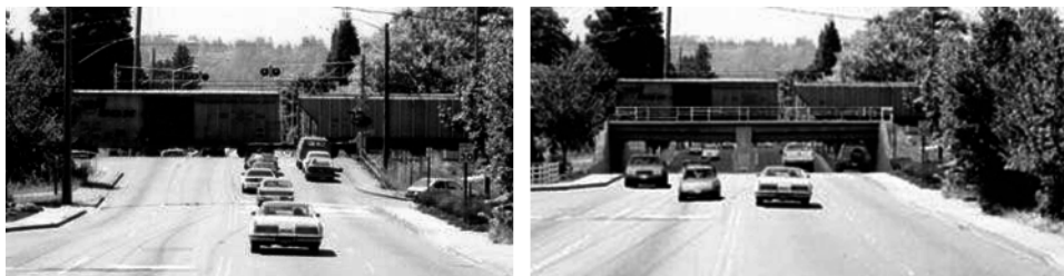
Figure 5: At-Grade Rail Crossing Near Ports of Seattle/Tacoma—before and after Construction of Overpass
