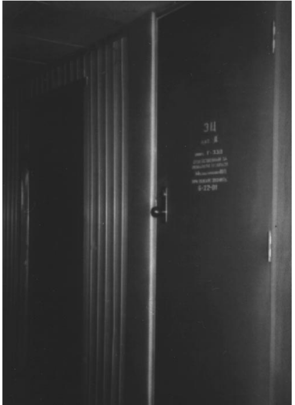
Figure III.5: Prototype Metal Fire Door to Be Installed at Smolensk Nuclear Power Plant
