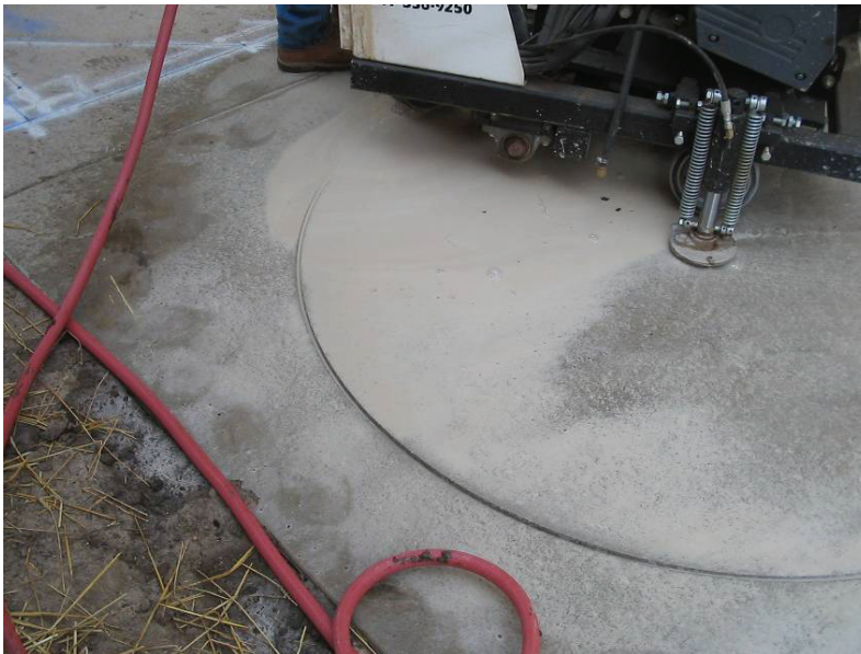
Figure 5-43. Round sawcut in process.
