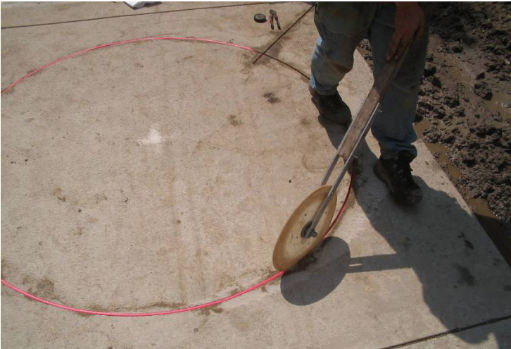
Figure 5-48. Firmly seating backer rod material over loop wire.
