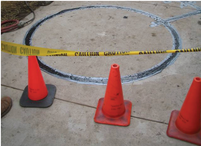
Figure 5-52. Isolation of affected area to allow sealant to dry.
