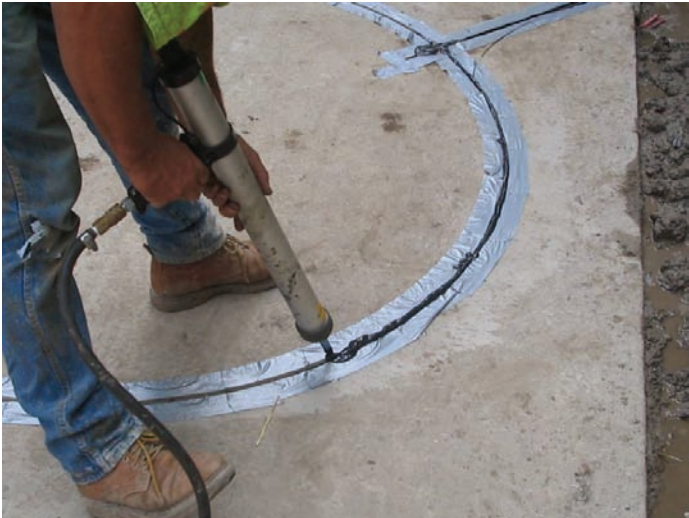
Figure 5-50. Placing sealant in sawcut.
