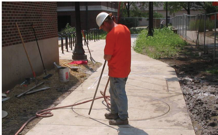
Figure 5-45. Blowing out debris from sawcut.
