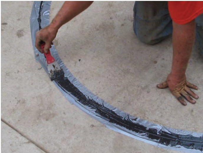
Figure 5-51. Removing excess sealant.
