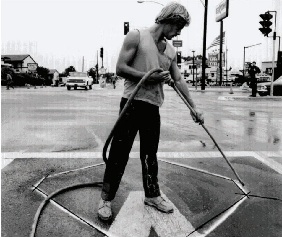
Figure 5-4. Pavement blow drying.
