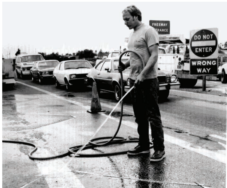
Figure 5-3. Pavement washing.
