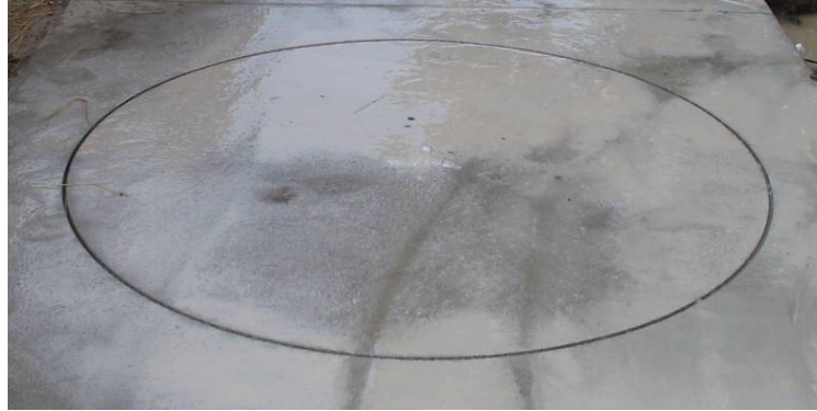
Figure 5-44. Completed round sawcut.
