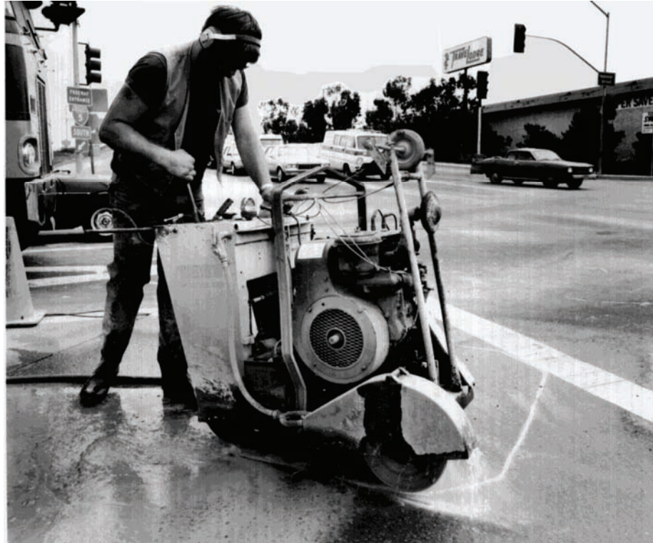
Figure 5-2. Loop sawcut process.
