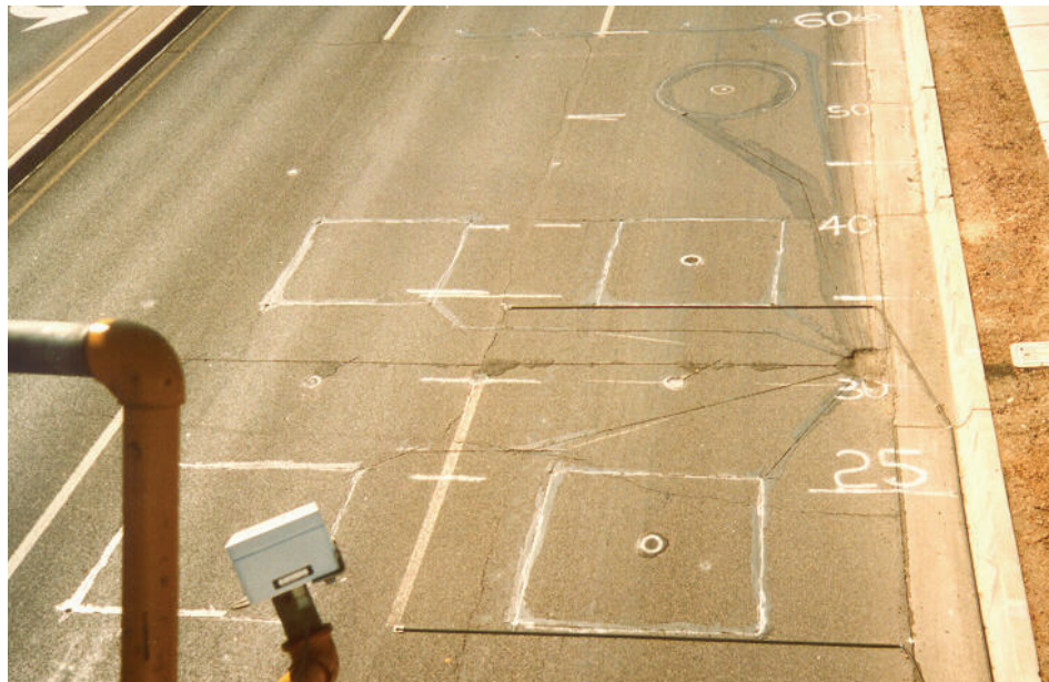
Figure 5-59. Down-lane road surface dimensions marked with paint as used for sensor evaluation and performance comparison.
