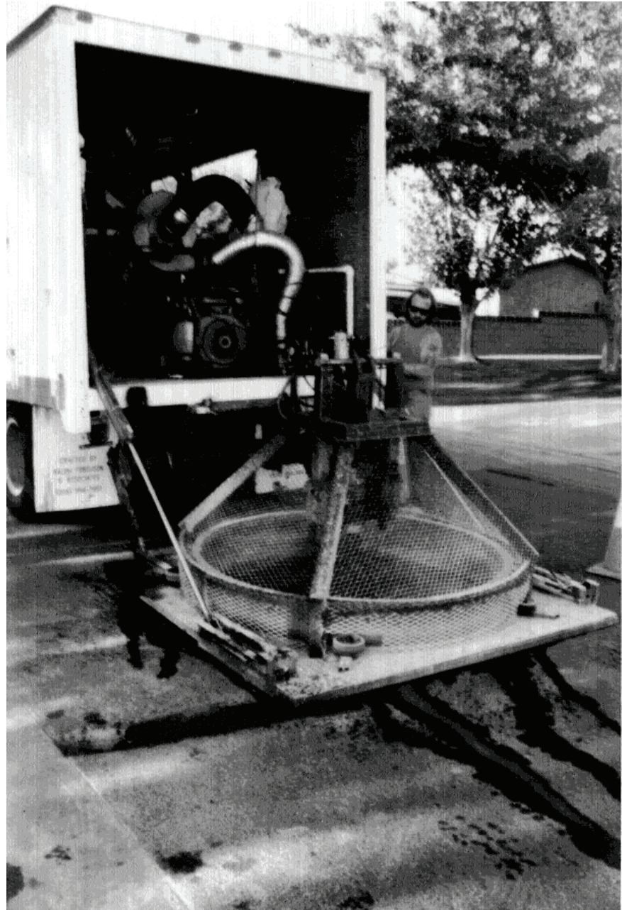
Figure 5-39. Roadway installation of round loops—cutting loop circle.
