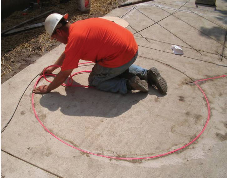
Figure 5-47. Inserting backer rod material over loop wire.
