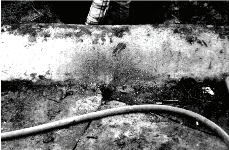
Figure 5-20. Entry hole for curb crossing installations.
