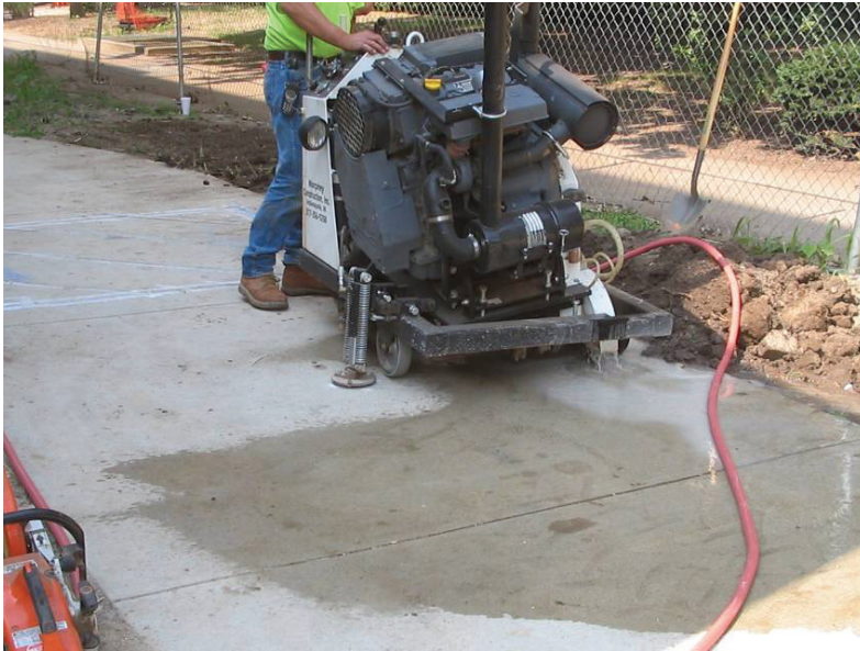
Figure 5-42. Round loop saw at beginning of installation process.
