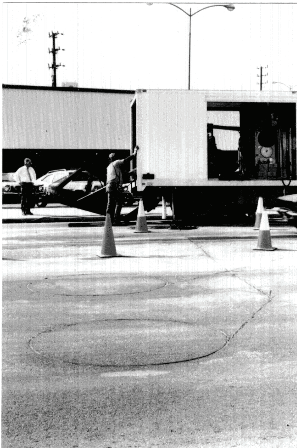
Figure 5-41. Roadway installation of round loops—completed installation.
