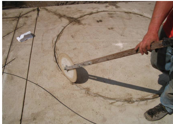
Figure 5-46. Firmly seating loop wire in sawcut with rolling-blade tool.
