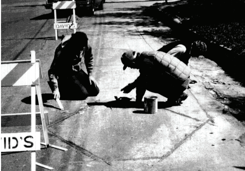
Figure 5-30. Finishing sealant application.
