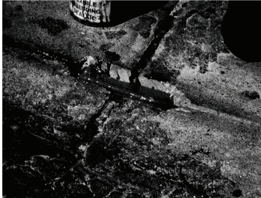
Figure 5-15. Crossing pavement joints using rigid tubing.
