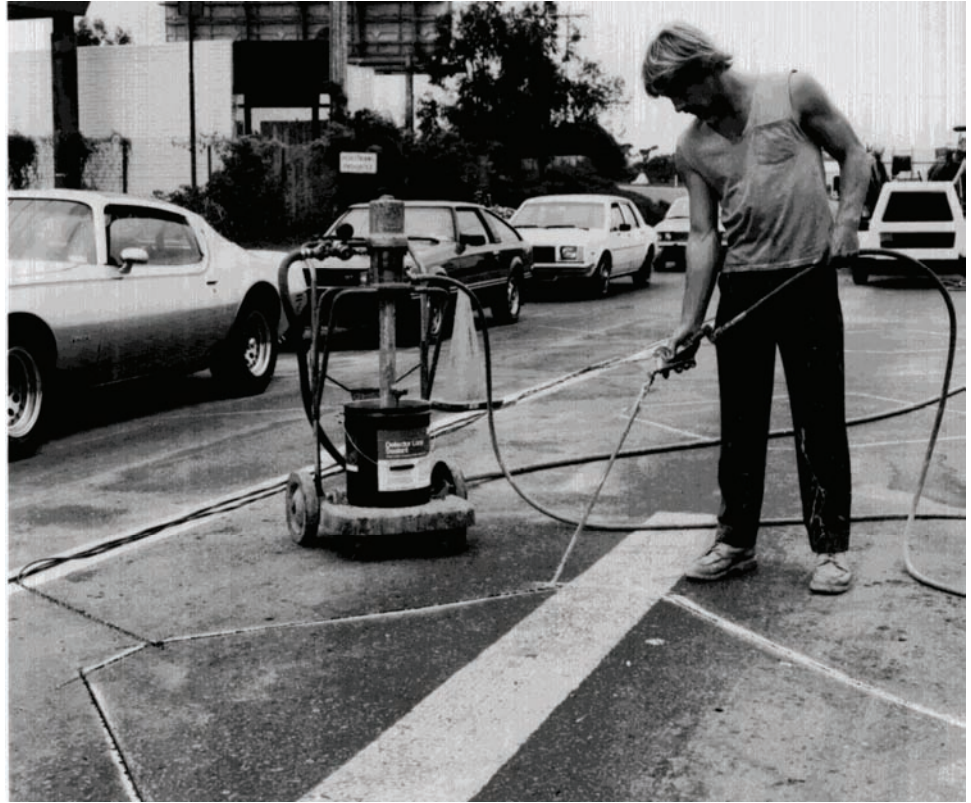
Figure 5-6. Inserting loop sealant.
