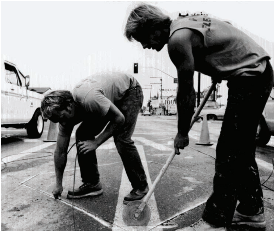
Figure 5-5. Pressing in wire and backer rod.
