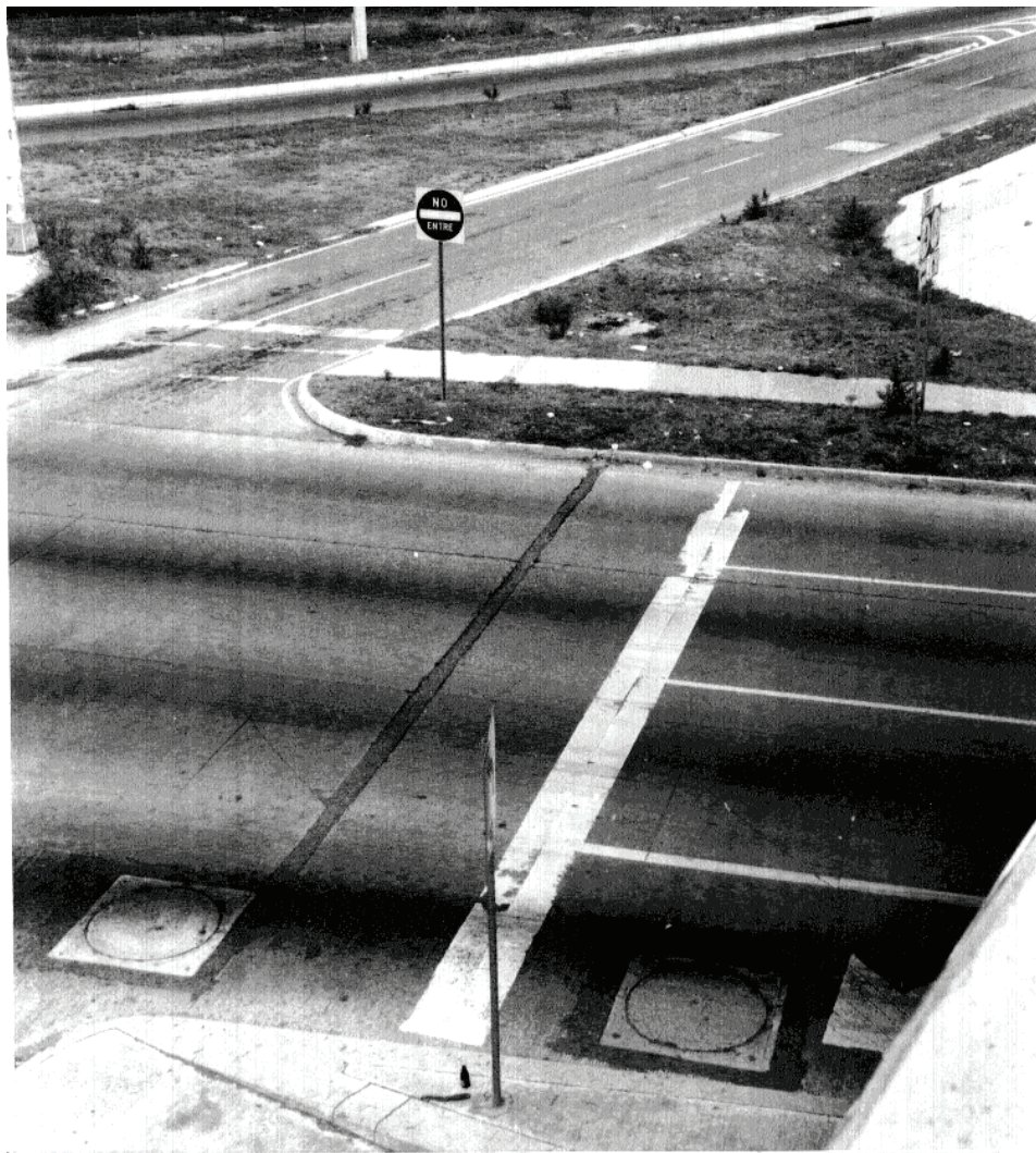
Figure 5-38. Slab-loop installations.
