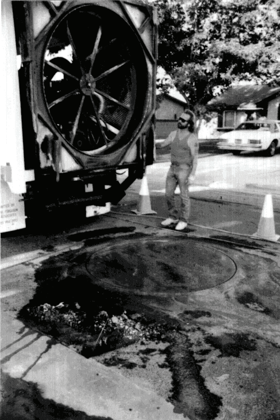
Figure 5-40. Roadway installation of round loops—retraction of saw.
