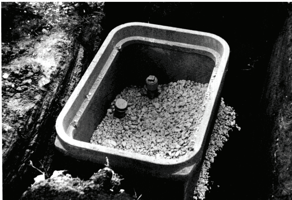
Figure 5-24. Standard pull box.
