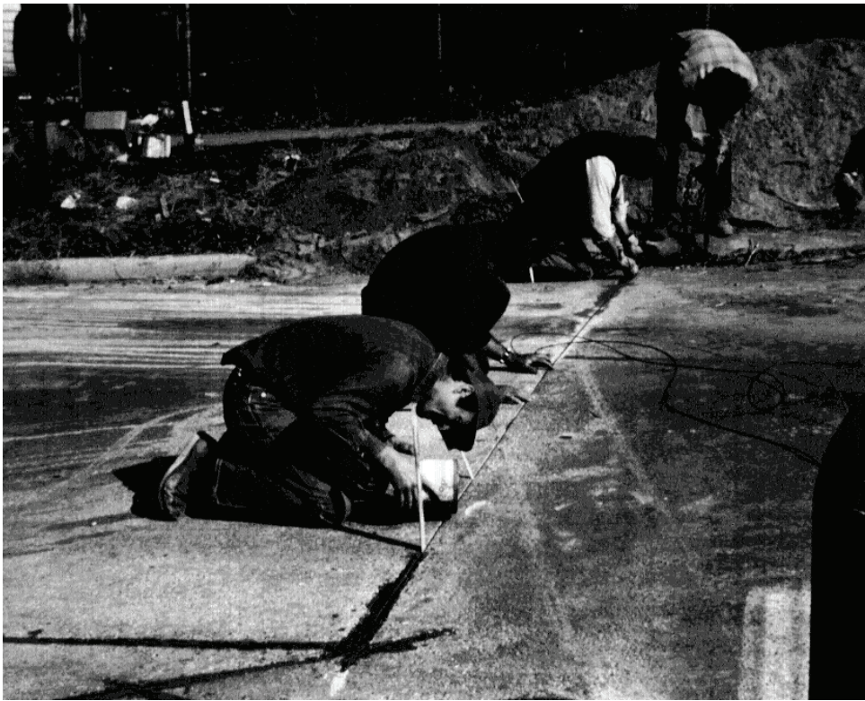
Figure 5-29. Crew applying sealant by hand.
