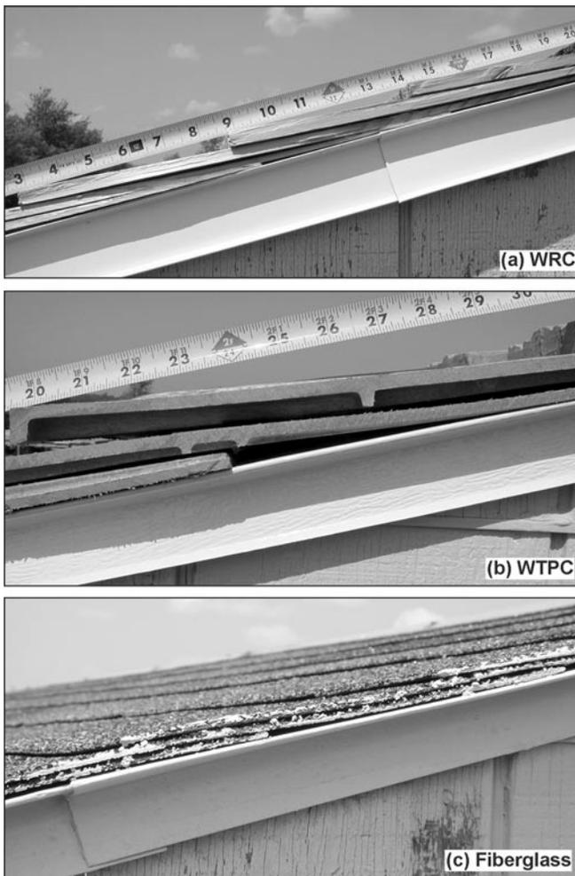
**Figure 2—Side view of installed shingles: (a) western redcedar (WRC), (b) wood–thermoplastic composite (WTPC), and (c) fiberglass.**
