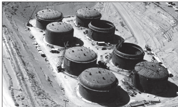
Double-Shell Tank Farm under Construction at Hanford
