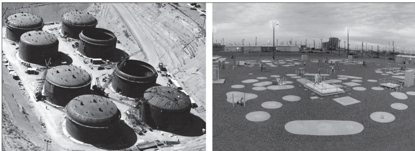
Figure 1: Double-Shell Waste Tanks under Construction and Completed Tank Farm at DOE's Hanford Site
