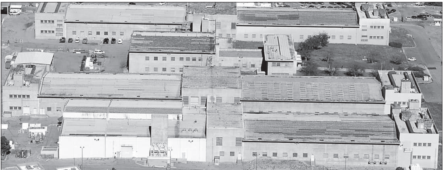
Figure 2: LANL's Chemistry and Metallurgy Research Facility
