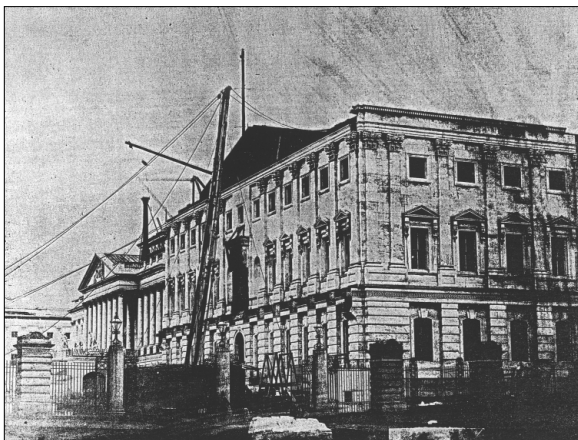
View of the north wing of the Capitol under construction, ca. 1856
