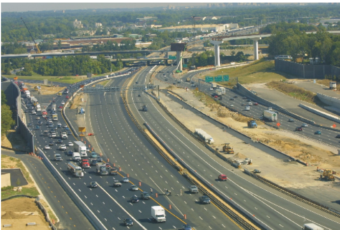
The Springfield Interchange in suburban Washington, D.C. has become one of the most costly highway projects in the country.
