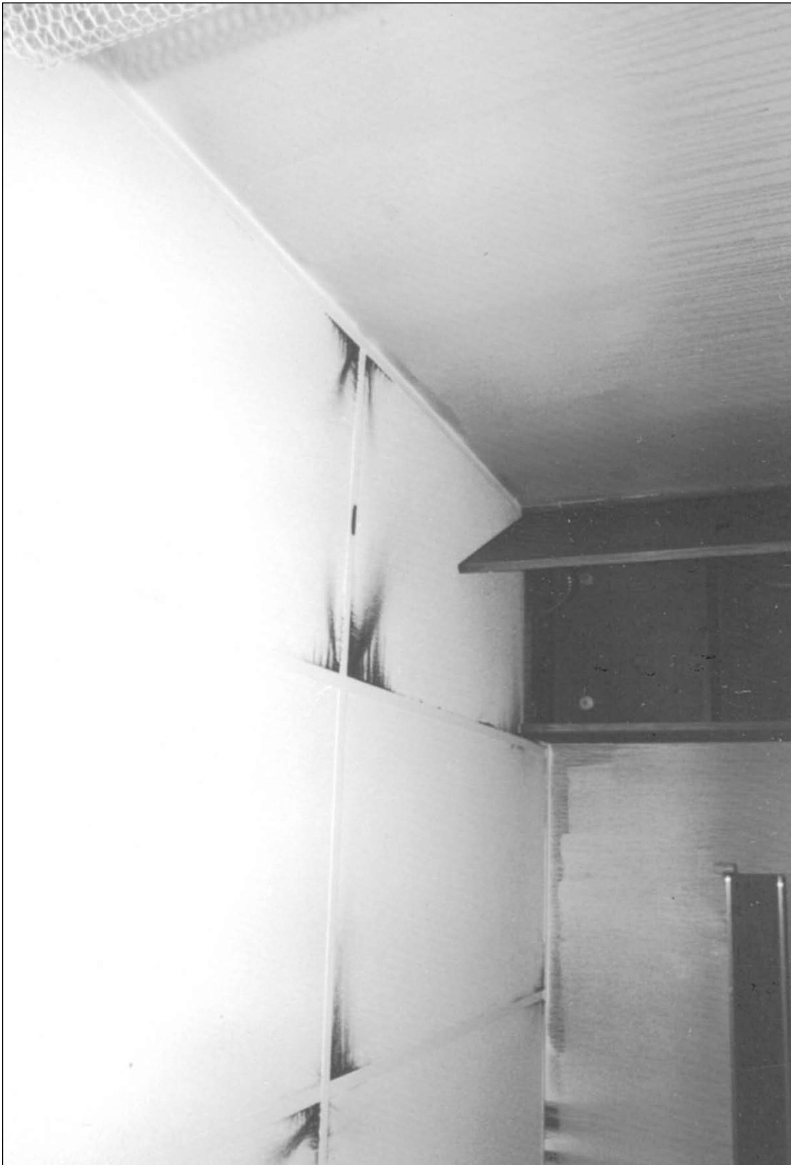
Smoke streaks on the ceiling indicate that smoke was entering the rooms adjacent to the fire room through the ceiling suspension system.
