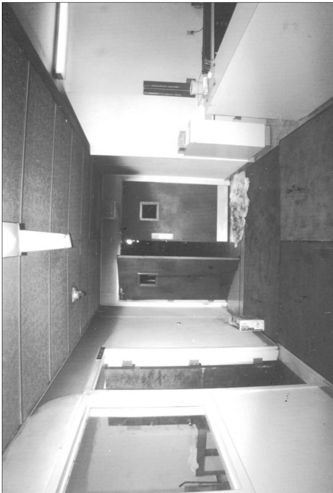
This photo looks down toward the south corridor with the nurses station on the right. The self-closing smoke control doors contained the bulk of the smoke and heat conditions to the corridor of origin, but some smoke escaped into the nurses station area as victims were evacuated through the doors.
