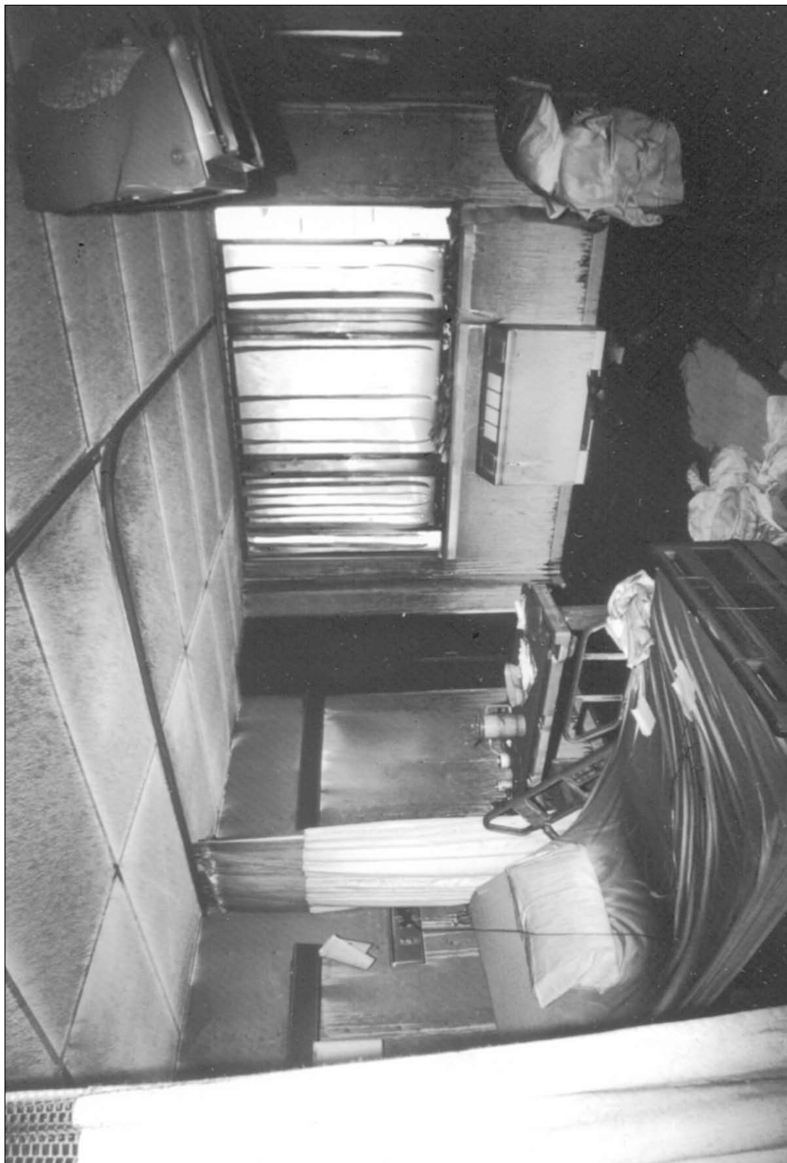
Room 421 which was located on the south corridor suffered heavy smoke damage. Nurses closed the door to this room, however, investigators believe the patient opened the door while attempting to escape. The patient was found lying in the doorway by the firefighters.
