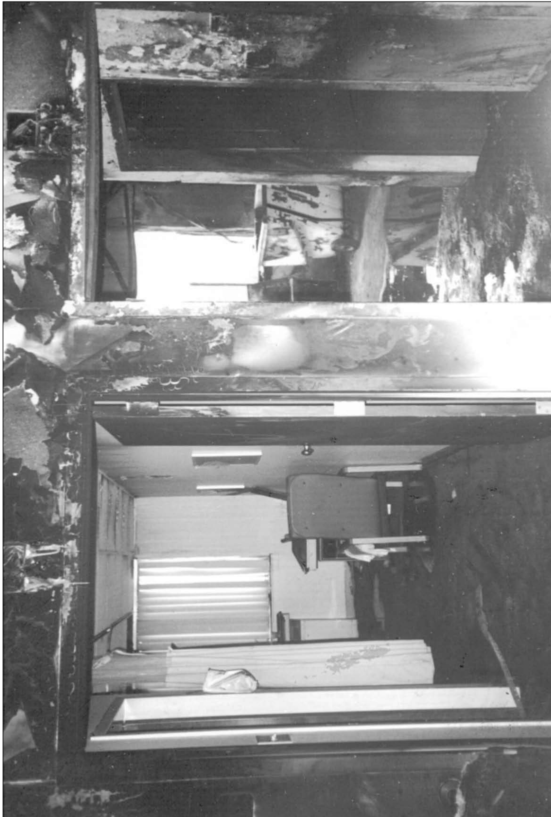
This photo shows the heavy damage to the fire room, Room 418 (on the right), and the adjacent room, Room 419 (on the left). Nurses closed the door to Room 419, but heavy smoke infiltrated the room through the suspended ceiling and cracks around the edges of the door. The patients in both of these rooms died.
