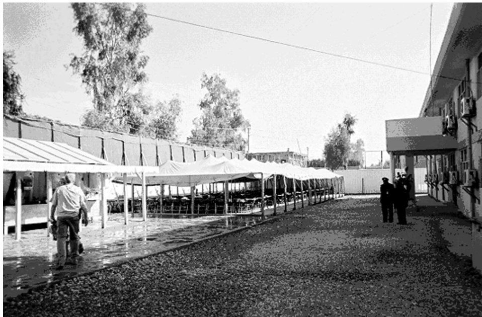
Figure 5: Police Regional Training Center in Jalalabad—Dining Facility and Classroom Building
