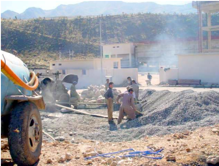
Figure 11: Oil for Food Program Funded the Construction of a Water Station in Northern Iraq
