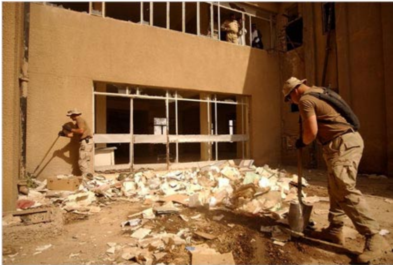
Figure 8: U.S. Navy Seabee Engineers Refurbishing the Al Nasiriyah Police Headquarters Building
