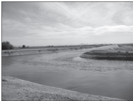
Source: GAO. Concrete-lined Irrigation Canal
