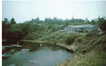
Figure 4. Kalaloch Lodge in Olympic National Park, Wash., is threatened by erosion. Long-term plans call for moving the lodge back from the cliff edge. Photograph by Erika Hammar-Klose, USGS.
