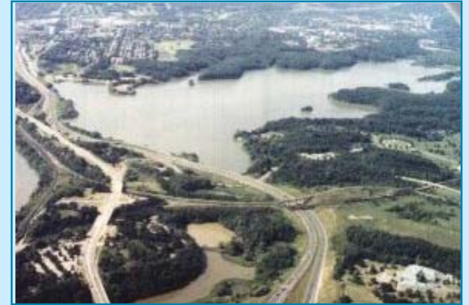
Credit: Bay Area Restoration Council
