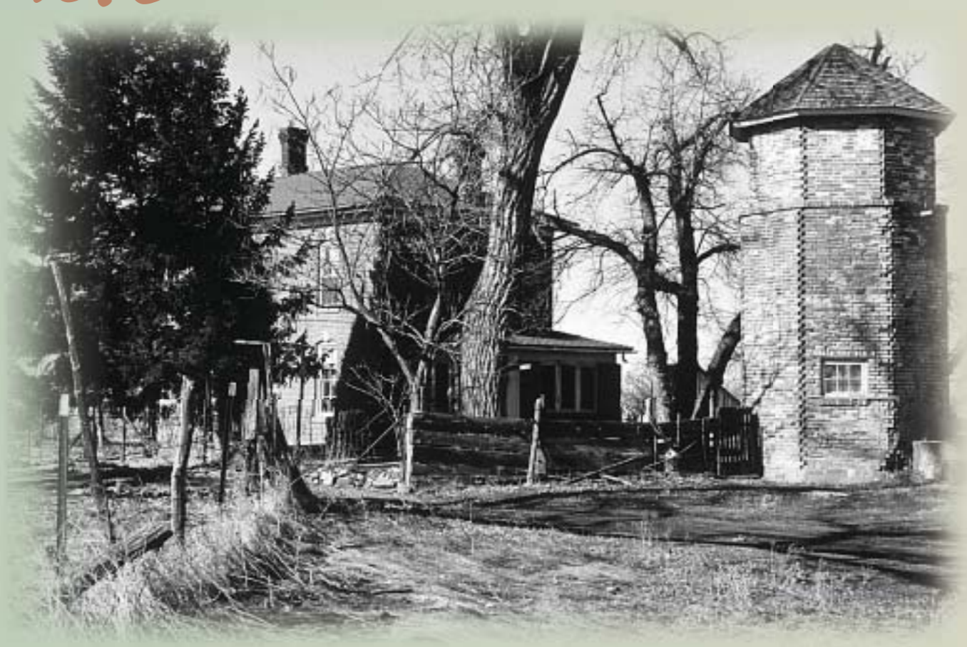
Figure 5. The Lee residence of Wheatridge, Colorado, built in 1873. (Photograph by D.L. Jarrett in 1961, courtesy Colorado Historical Society, Negative no. 38,764.)
