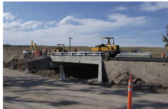
Another lift of HBP was placed before opening the road to traffic Sunday at 5PM.
