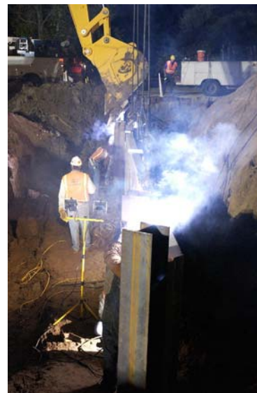
The hidewall is welded to the previously driven piles.
