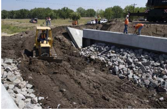
Rip-rap was placed concurrently with the flowfill and partially buried
