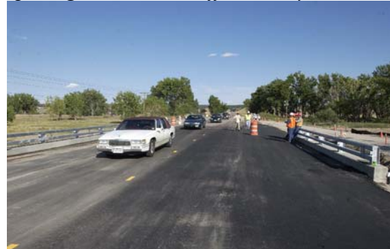
Another lift of HBP was placed before opening the road to traffic Sunday at 5PM.
