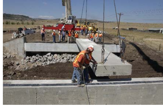
The first girder was placed mid-morning.
