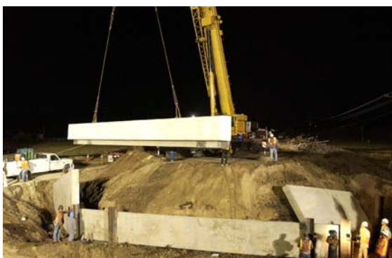
The abutment cap is brought in to complete the abutment.
