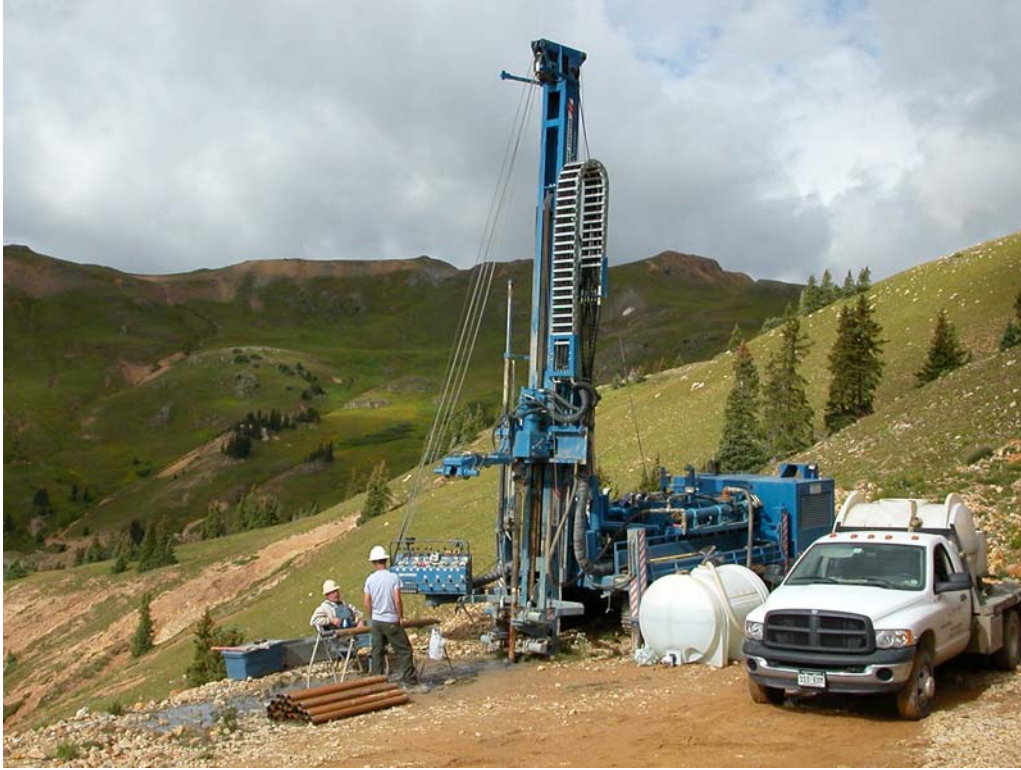
Figure 2. Boart Longyear Delta Base 540 drilling rig operated by Spectrum Exploration at upper elevation hole in Prospect Gulch.
