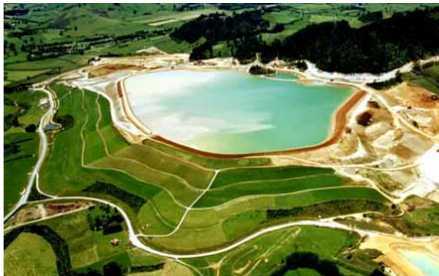
Figure 5. Tailings storage facility at the Martha Mine near Waihi, New Zealand, nearing its final height. This aerial photograph, which was taken in early 2000, shows the embankment structure. The lower slopes have been rehabilitated. The impoundment where tailings are deposited as a slurry can be clearly seen as can the light-colored tailings beach at the far left end of the pond (Waihi Gold Mining Company Limited, undated).
