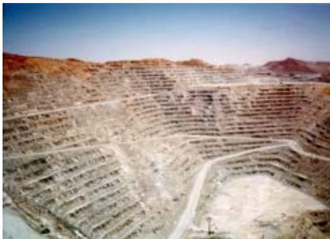
Figure 1. Phelps Dodge Mining Company's Sierrita open pit copper mine in Sierrita, Arizona. (Arizona State Mine Inspector's Office, 202)
