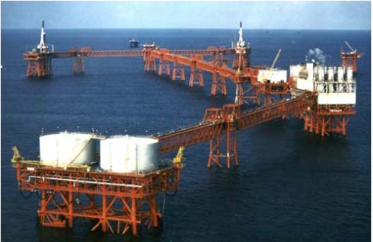
Figure 5. Photograph that shows the last sulfur mine in the United States, Freeport-McMoRan Sulphur Inc.'s Main Pass Mine, that closed in August 2000. Located about 51 kilometers (32 miles) offshore, it was the largest structure in the Gulf of Mexico with its platform extending more than 1.6 kilometers (more than 1 mile). Photo courtesy of Freeport McMoRan Sulphur Inc.
