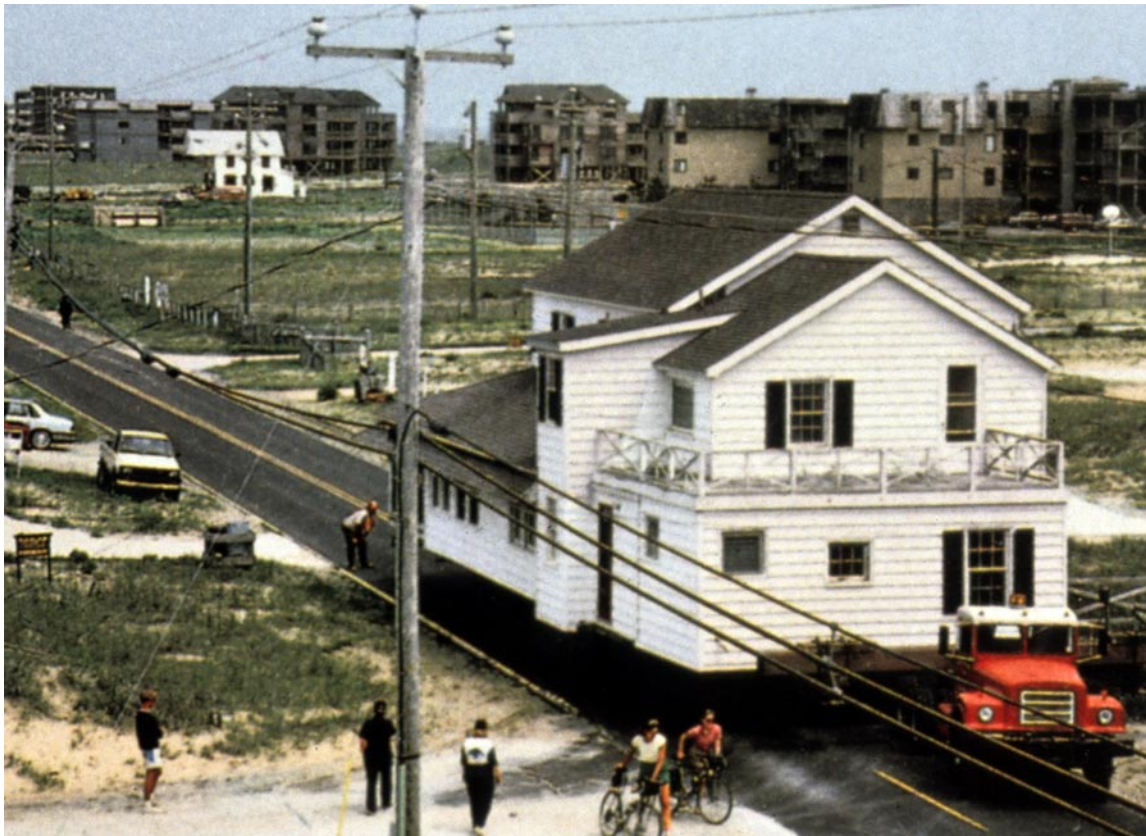
Figure 20. Lateral relocation of a beach house in North Carolina is an example of retreat from the eroding shore. Photo source is unknown.
