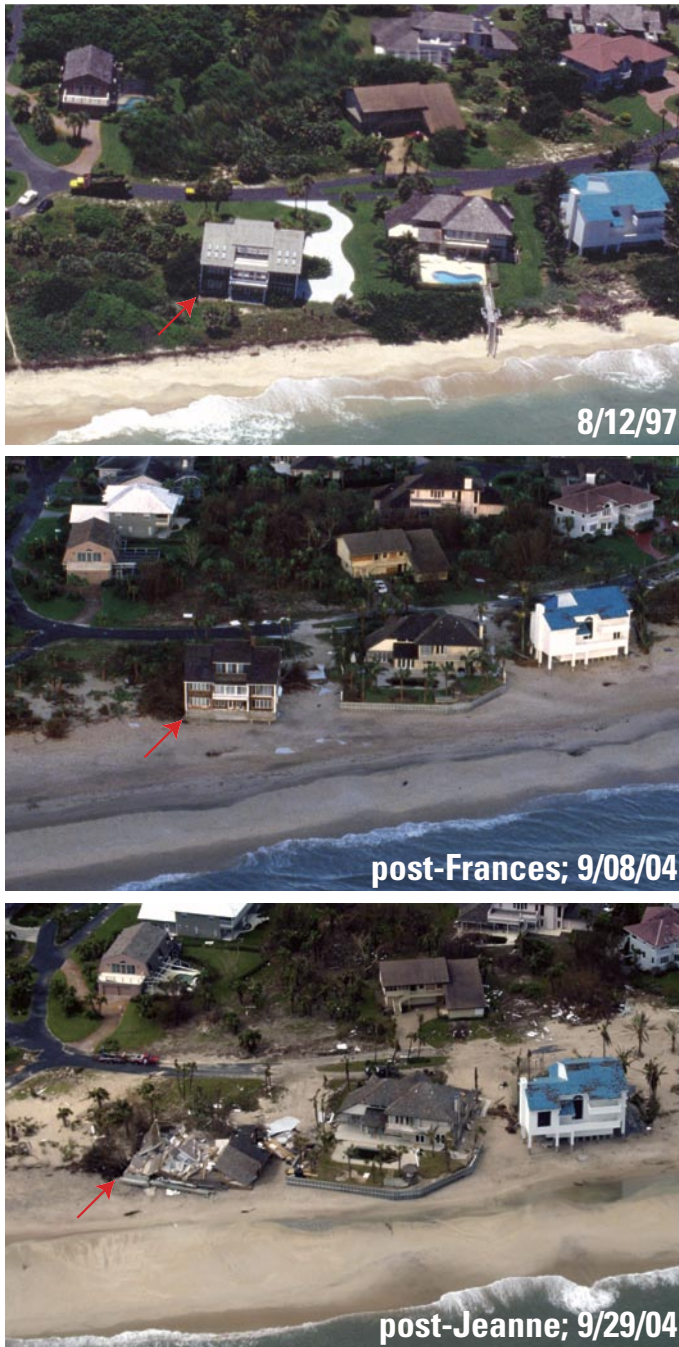
Figure 13. Erosion and property damage near Floralton Beach, Florida caused by Hurricanes Francis and Jeanne in 2004.
