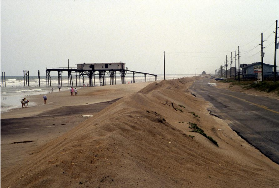
Figure 12. Erosion of the Atlantic shore can destroy roads and eliminate the beach. This example at Topsail Island, North Carolina, shows the effects of long-term erosion and efforts to protect the highway.
