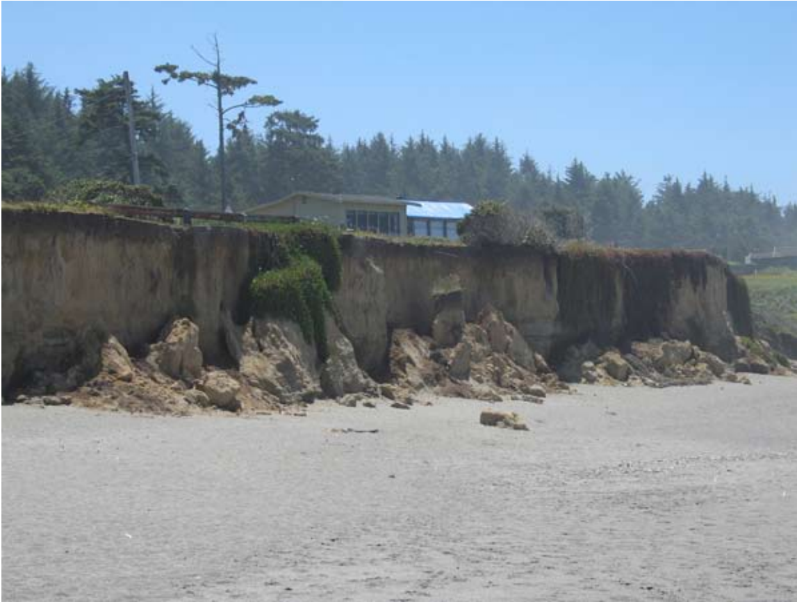
Figure 16. Bluff erosion at Big Lagoon Beach after an El Niño storm in the winter of 1983 (photo: Gary Griggs, UCSC).
