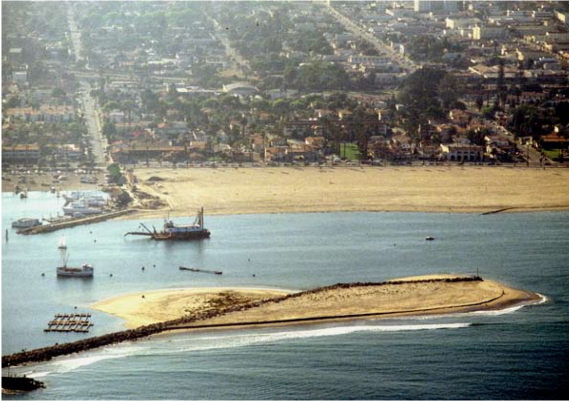
Figure 36. Dredging of spit at Santa Barbara Harbor. Dredged material is placed down-drift of the harbor where it replenishes East Beach, which accreted more than 6.0 m/yr from the 1970s to 1990s. (photo: Copyright © 2002-2005 Kenneth & Gabrielle Adelman, California Coastal Records Project, www.californiacoastline.org).
