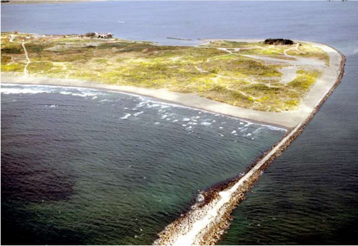
Figure 18. Spit and jetty on north side of Humboldt Bay Harbor in photograph taken in June 1987. North is to the left in the photograph. (photo: Copyright © 2002-2005 Kenneth & Gabrielle Adelman, California Coastal Records Project, www.californiacoastline.org )
