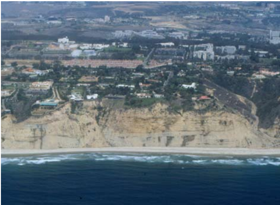
Figure 42. Narrow beach fronting tall coastal bluffs at Torrey Pines City Beach. The short-term beach erosion rates are high in this area (photo: Gary Griggs, UCSC).
