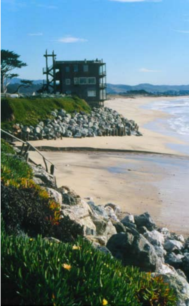
Figure 26. A riprap revetment protects an apartment building that overlooks a narrow beach near Pillar Point Harbor in a photograph taken in February, 2002. Note that the beach (background) with no revetment is much wider (photo: Gary Griggs, UCSC).
