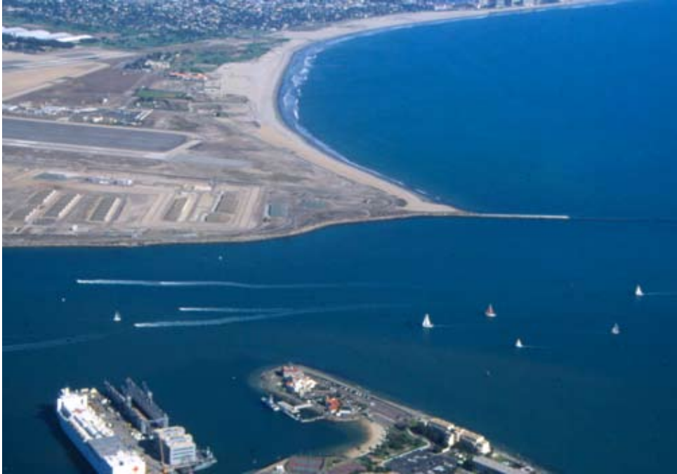
Figure 44. Oblique aerial photograph of Zuniga Point and breakwater at the entrance to the San Diego Harbor (photo: Cheryl Hapke, USGS).
