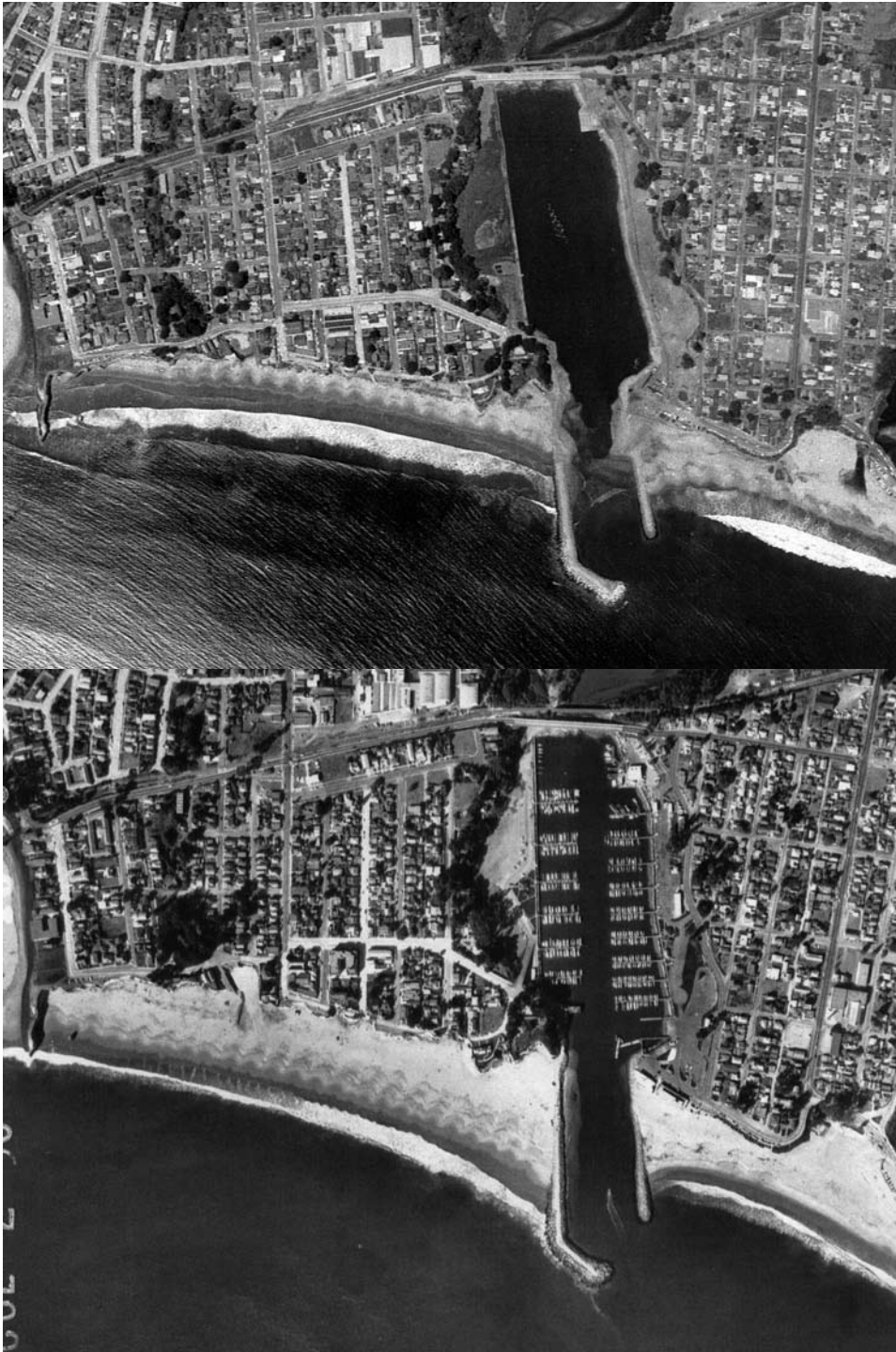
Figure 28. Aerial photographs of the Santa Cruz Yacht Harbor show the impoundment of sand against the constructed jetties. The top photo is from 1963, one year after the jetties were constructed. The bottom photo is from 1987, and shows a now wide, sandy beach (Seabright Beach) on the upcoast side of the jetty (photos: Santa Cruz Harbor Master's Office).
